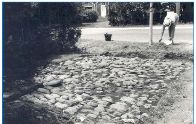
Blacksmith floor - Myrtle, Ontario
